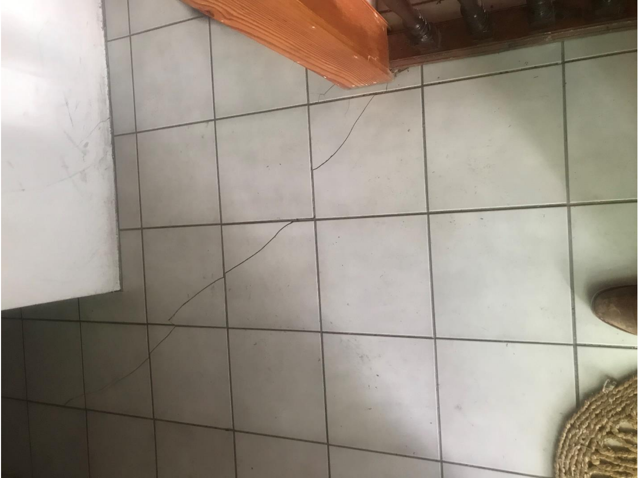
Figure 9: Showing crack through existing tiles
