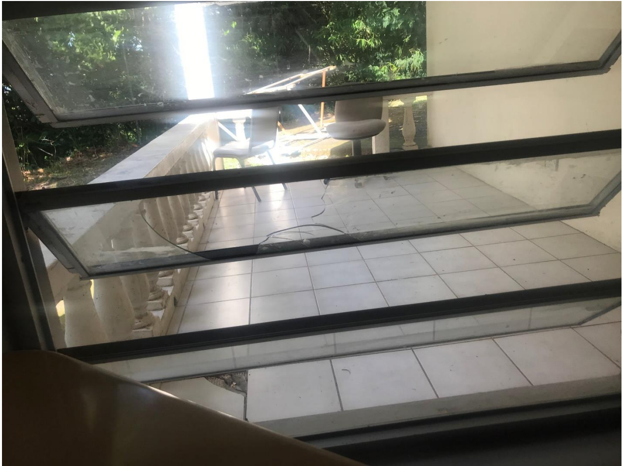
Figure 22: Showing broken glass on existing window
