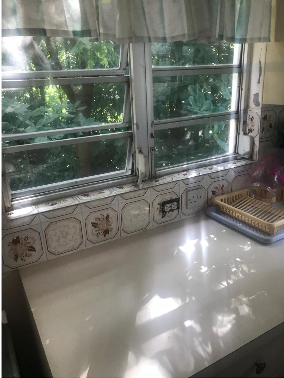
Figure 20: Showing window operator missing
