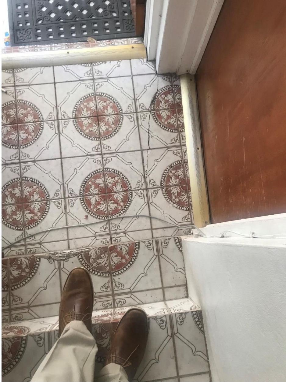
Figure 15: Showing crack through existing tiles
