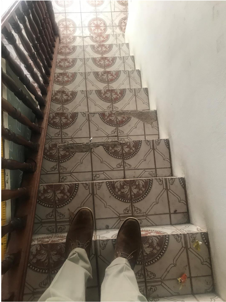
Figure 14: Broken tile on existing internal staircase
