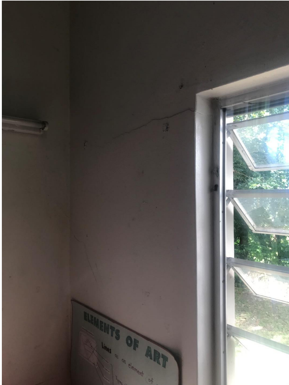
Figure 17: Showing crack on existing wall downstairs
