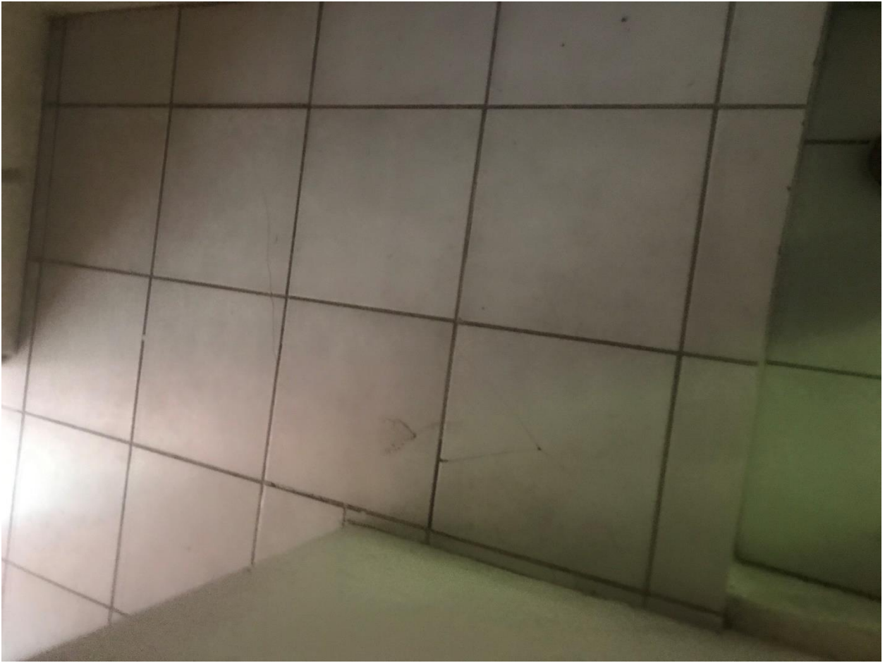
Figure 10: Showing crack through existing tiles
