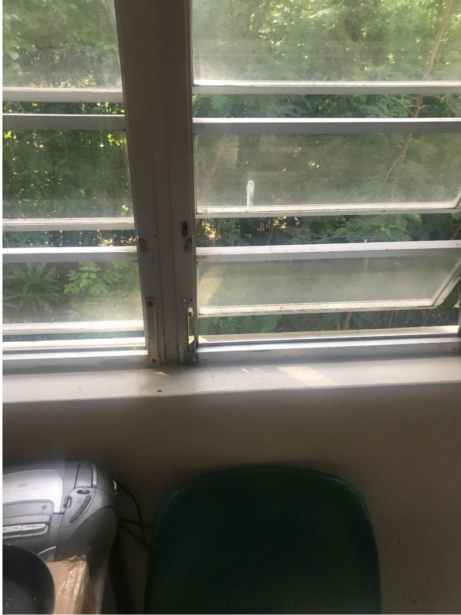
Figure 19: Showing window operator missing
