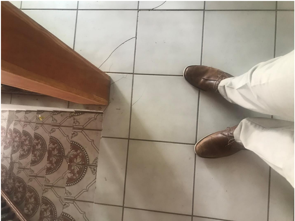
Figure 11: Showing crack through existing tiles
