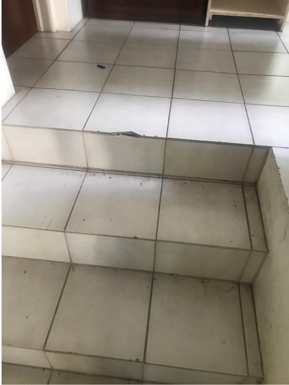
Figure 18: Showing chipped tile on the existing staircase downstairs
