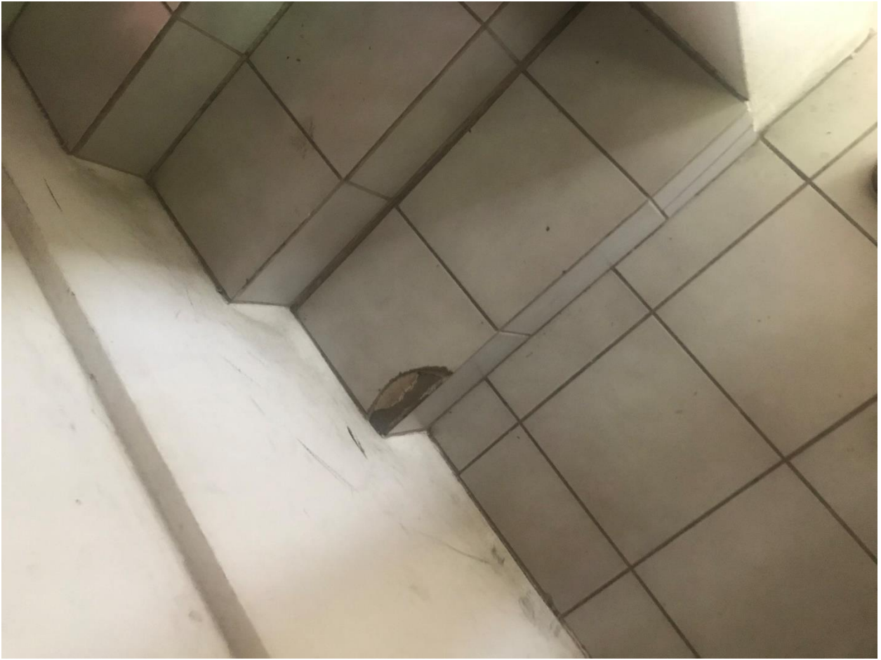
Figure 12: Showing a broken tile on the existing internal staircase
