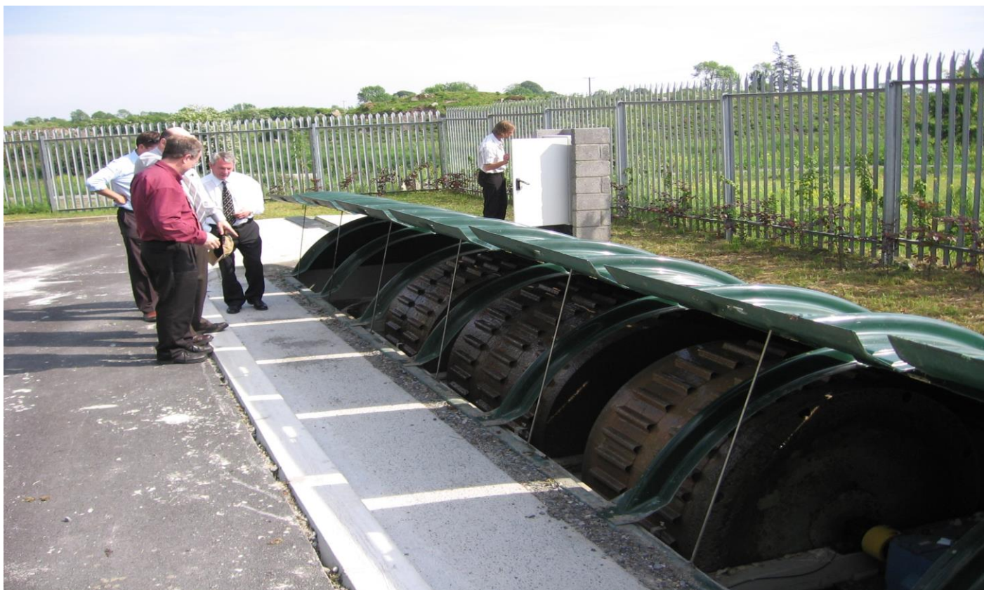
Figure 3: BMS BL3500 Blivet installed below ground
