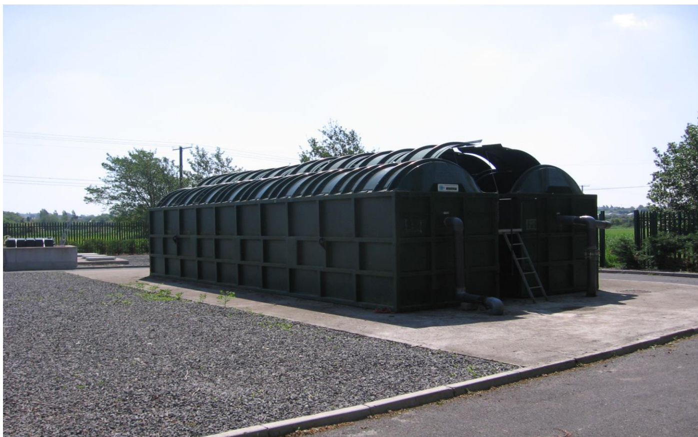
Figure 4: BMS BL4000 Blivet's installed above ground
