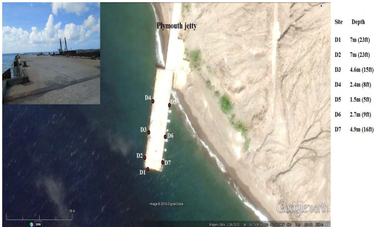
Figure 6.2: Plymouth Jetty Area (Inset: picture of jetty)
