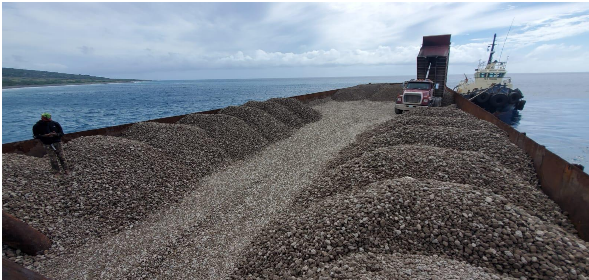
Material being loaded on a barge
