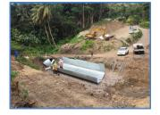
Despite these challenges a number of tasks were accomplished at the end reporting quarter. This includes (i) completion of the assembly of the bridge, (ii) backfilling of the bridge, (iii) 90% completion of the retaining walls and (iv) 50% completion of the drainage system. Despite the challenge of being six weeks behind the planned schedule, the project is deemed 70% completed at the end of this reporting period, with expenditure standing at EC\$0.88M.
