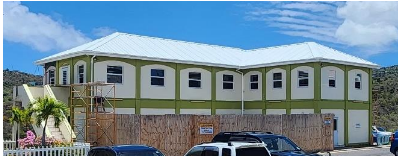
Court & Registry Building
