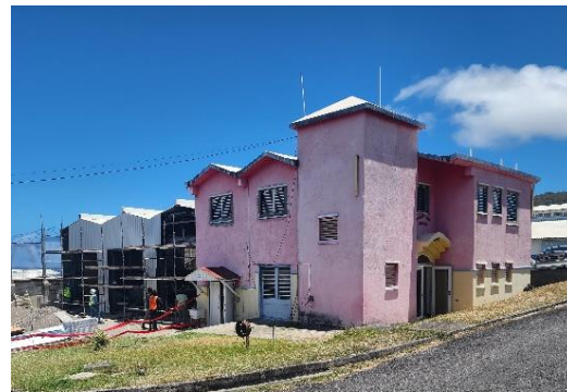
Fire Station Roof Repairs
