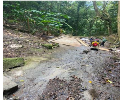
Fogarthy Springs: Catchment box top protecting springs from surface run-off.
