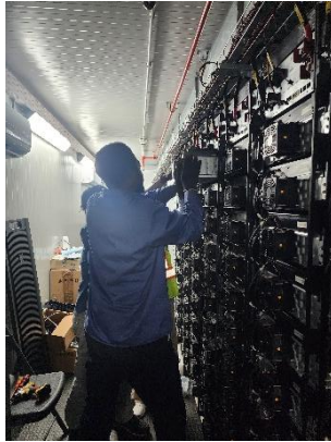
Look Out BESS Refurbishment
