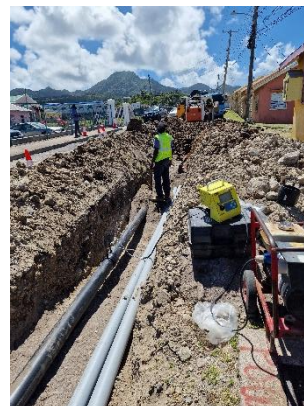
Look Water and Electricity Undergrounding
