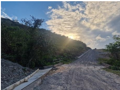
Garlin Hill Road Drainage
