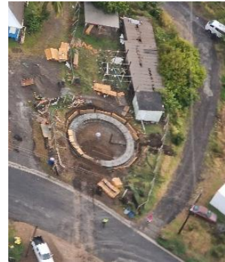
Davy Hill Reservoir Site
